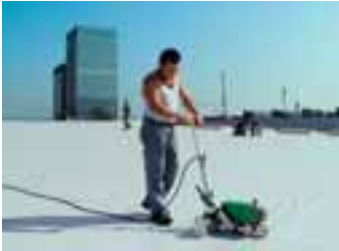
VARIMAT V used for overlap welding of plastic roofing membranes.
