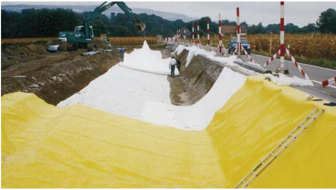
Geomembranes in road construction, Switzerland
