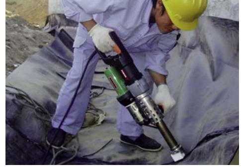
Thanks to its length, the FUSION 3 is particularly suitable for civil engineering applications.
