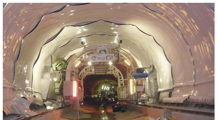
Tunnel construction in Germany
