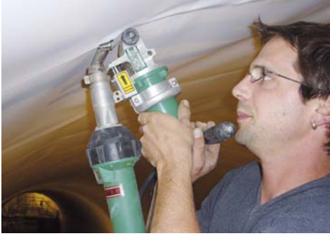
TRIAC DRIVE PID welding overhead in the tunnel construction.
